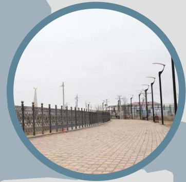
Shore protection in Kursai river, Kulsary city, Zhylyoi district
