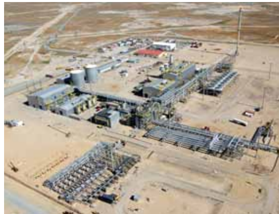
Sour Gas Injection facilities
